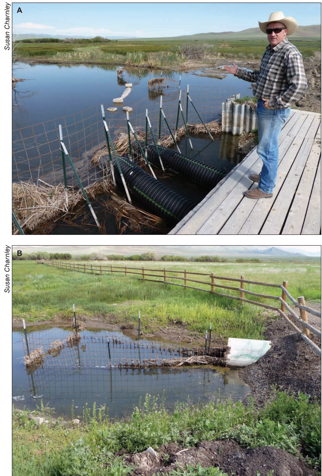
Figure 11—Some ranchers have begun to install devices that help mitigate the negative impacts of beaver: (A) A flow device on the Winecup Gamble Ranch prevents beaver from blocking water flowing under a bridge and flooding a road crossing; (B) A “beaver deceiver” prevents beavers from blocking a road culvert.
